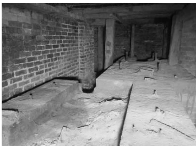
Fig 15. Beneath sawing area to north
