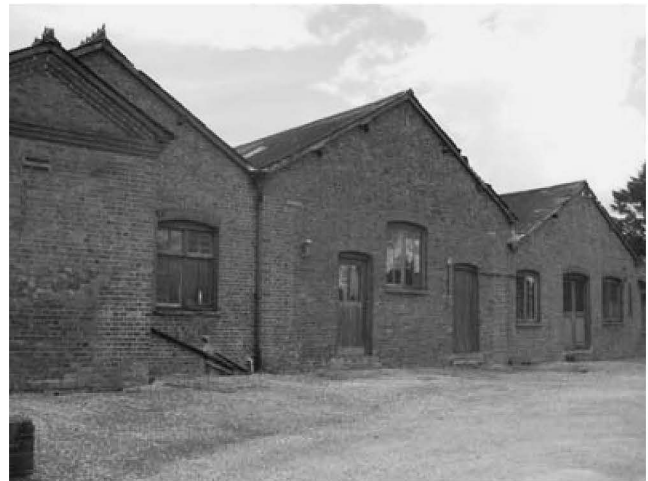
Fig 12. Building E - main workshops, south elevation.
